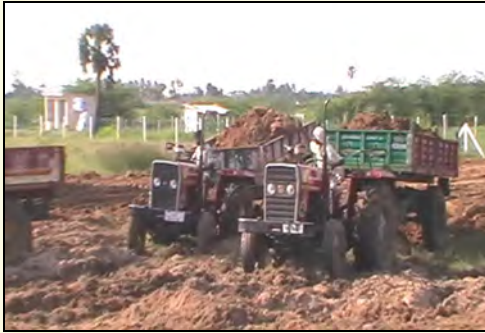
Continuation of Leveling Work
