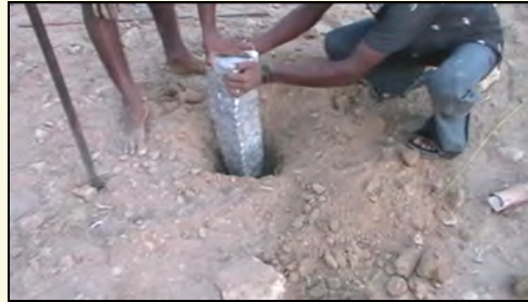
Fixing Plot Boundary Stone
