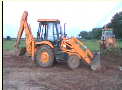
Continuation of Leveling Work
