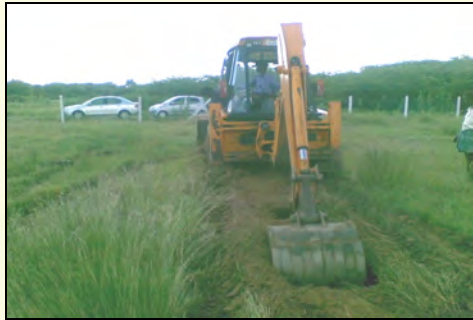
Excavator Involved in Leveling Work
